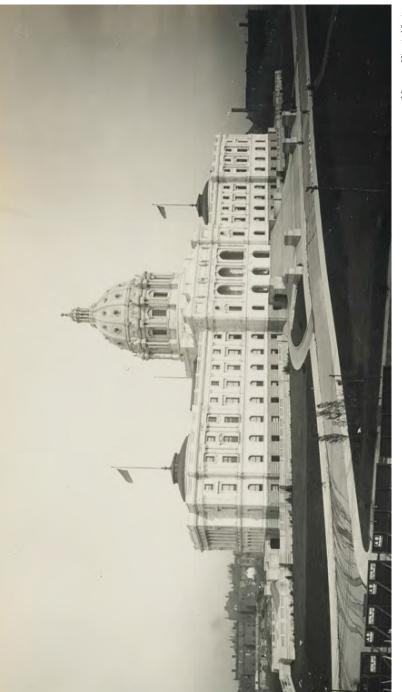
Shown is the Capitol in its completed state, except for the golden Quadriga. The Quadriga was placed in 1906, one year after the Capitol opened. The lower levels and stairs of the building (darker in color) were made of granite from central Minnesota. The remainder was marble quarried in Georgia and shipped to St. Paul. The photo also depicts Cass Gilbert's original vision, which inspired the Restoration plan, for the pedestrian promenade and landscaping.
