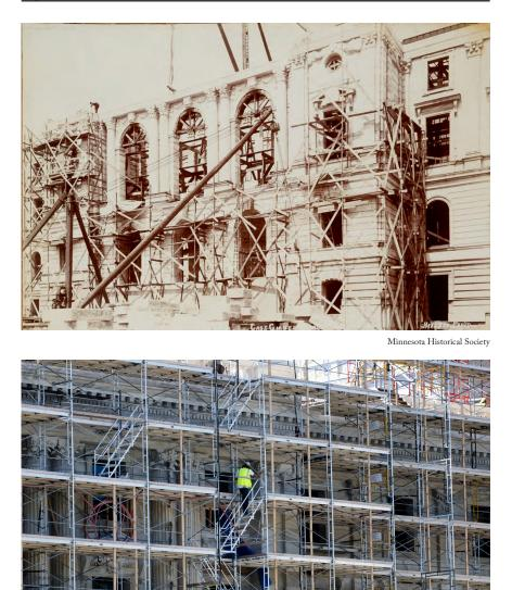
Scaffolding was installed on one face of the building at a time to allow for stone investigation, repair, and replacement work. While the materials have changed and safety has improved, the basic concept of scaffolding as the best way to affect exterior repairs remains the same today as it was over 100 years ago. Some records indicate that six people died on the jobsite during the original construction of the Capitol.
