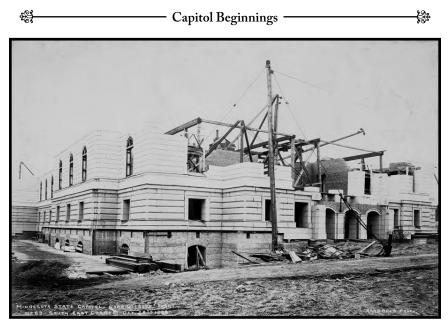
A photo captured on October 28, 1898 shows the exterior stone walls of the Capitol beginning to grow in height. The lower two levels were made of granite from Central Minnesota. The remainder was marble from Georgia.
